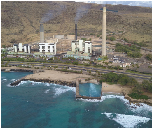
Figure 1: Kahe Power Plant (HECO)
